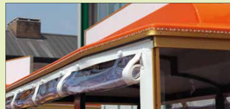
Decorative led lighting system around roof
