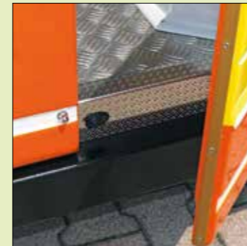
Electric door contacts (signalling any open doors)
